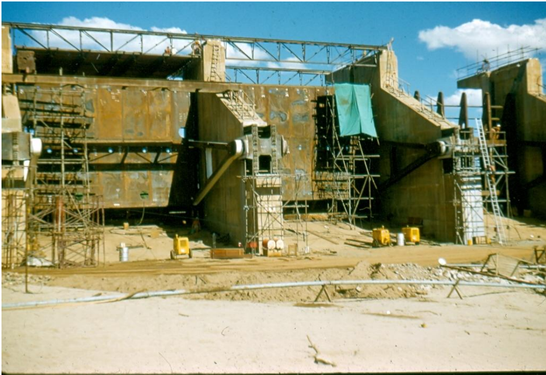
Radial gates 1, 2 & 3 progress
