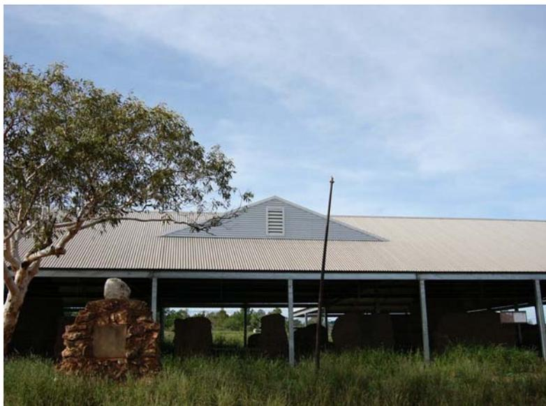
New gable, installed on the front elevation, 2006. The infill in the gable end has been duplicated in the two existing gables. The age of the tree in the photograph is unknown but, as can be seen from the photograph below, it has undergone little change since the 1940s. Photograph courtesy of Murray River North Pty Ltd.
